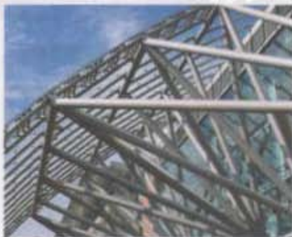
Steels have many uses in modern buildings
