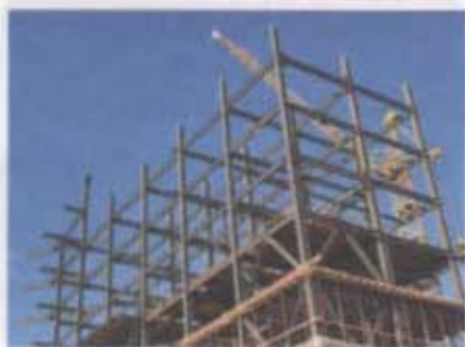
Steel girders are used in many buildings
