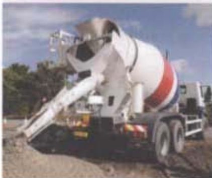
Concrete is mixed, poured and left to set
